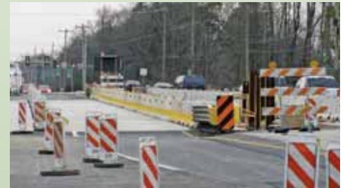
Photos of improvement projects at US 202 (DeKalb Pike)
